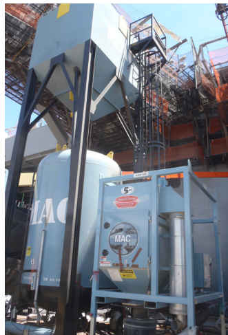
MAC dry blasting equipment on the job site.
